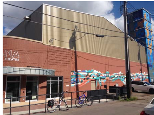
WEST FAÇADE OF COMPLETED BUILDING
