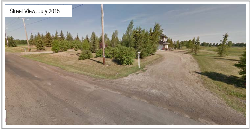
Figure 2. Street View Image of 15860 – 41 Avenue SW on 41 Avenue SW
