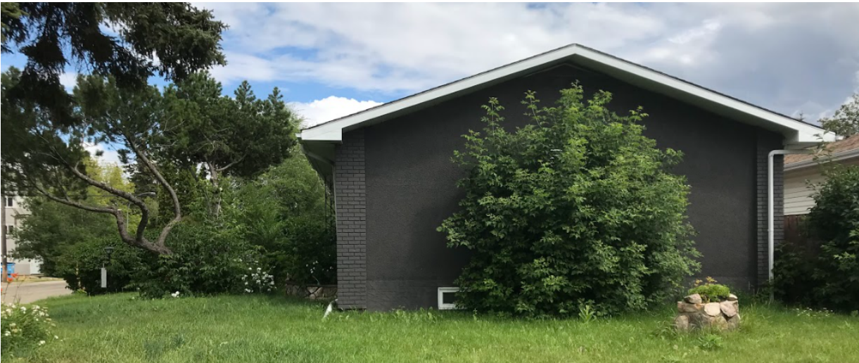
View of the site looking east from 150 Street NW.
