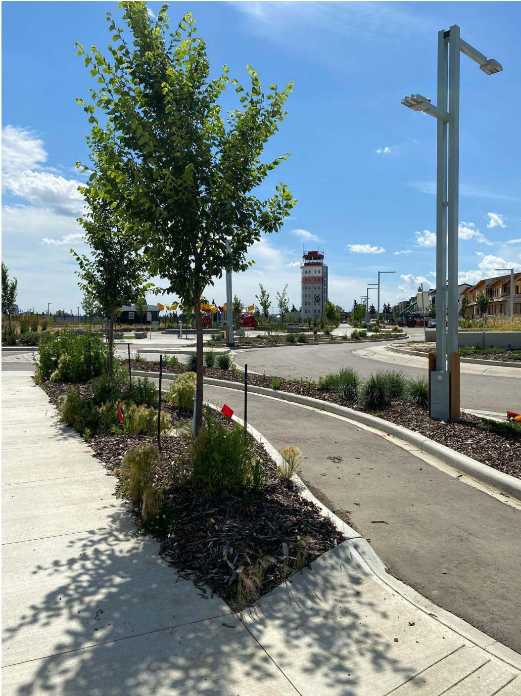
Custom street design including narrower roads, wider sidewalks, separated bike lanes and boulevard trees encourage active modes of transportation.
