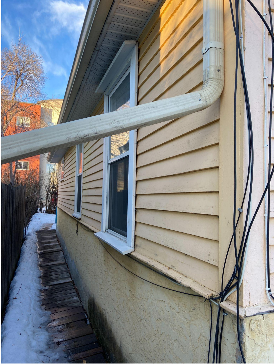
Detail of west elevation, looking north.
