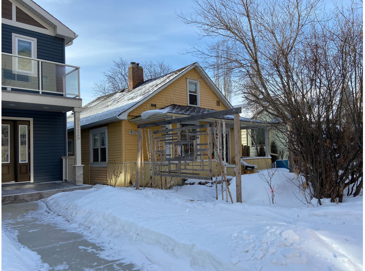
East and north (front) elevations, looking southwest.
