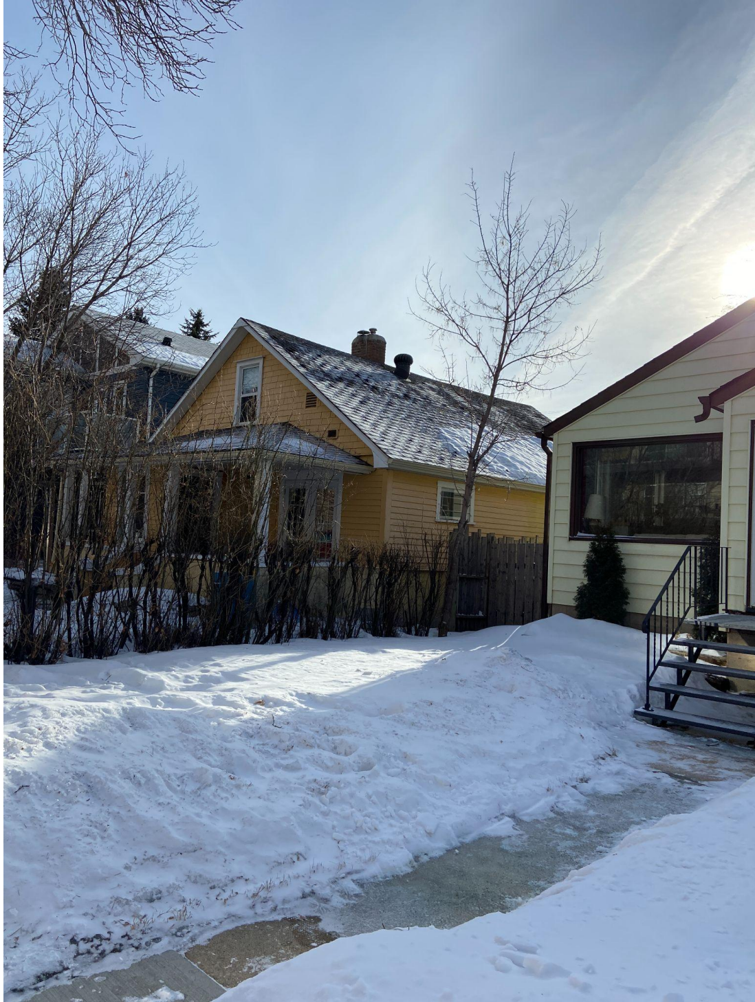
West and north (front) elevations, looking southeast.
