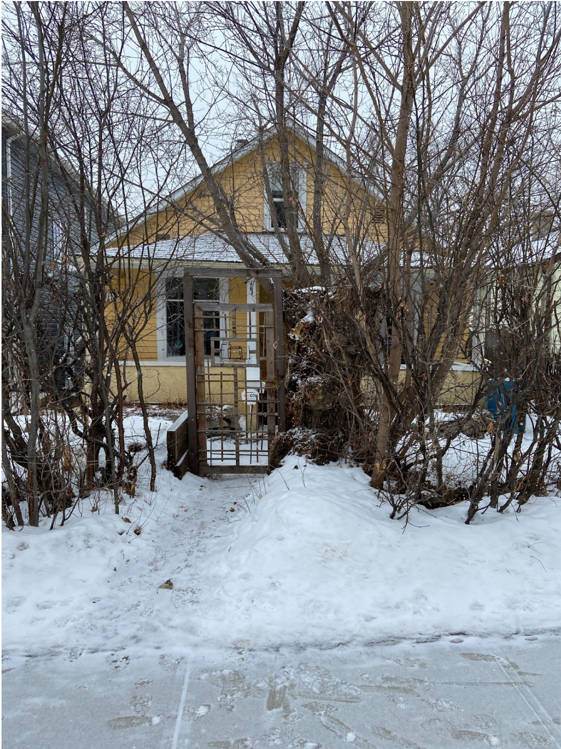
North (front) elevation, looking south from 84 Avenue NW.
