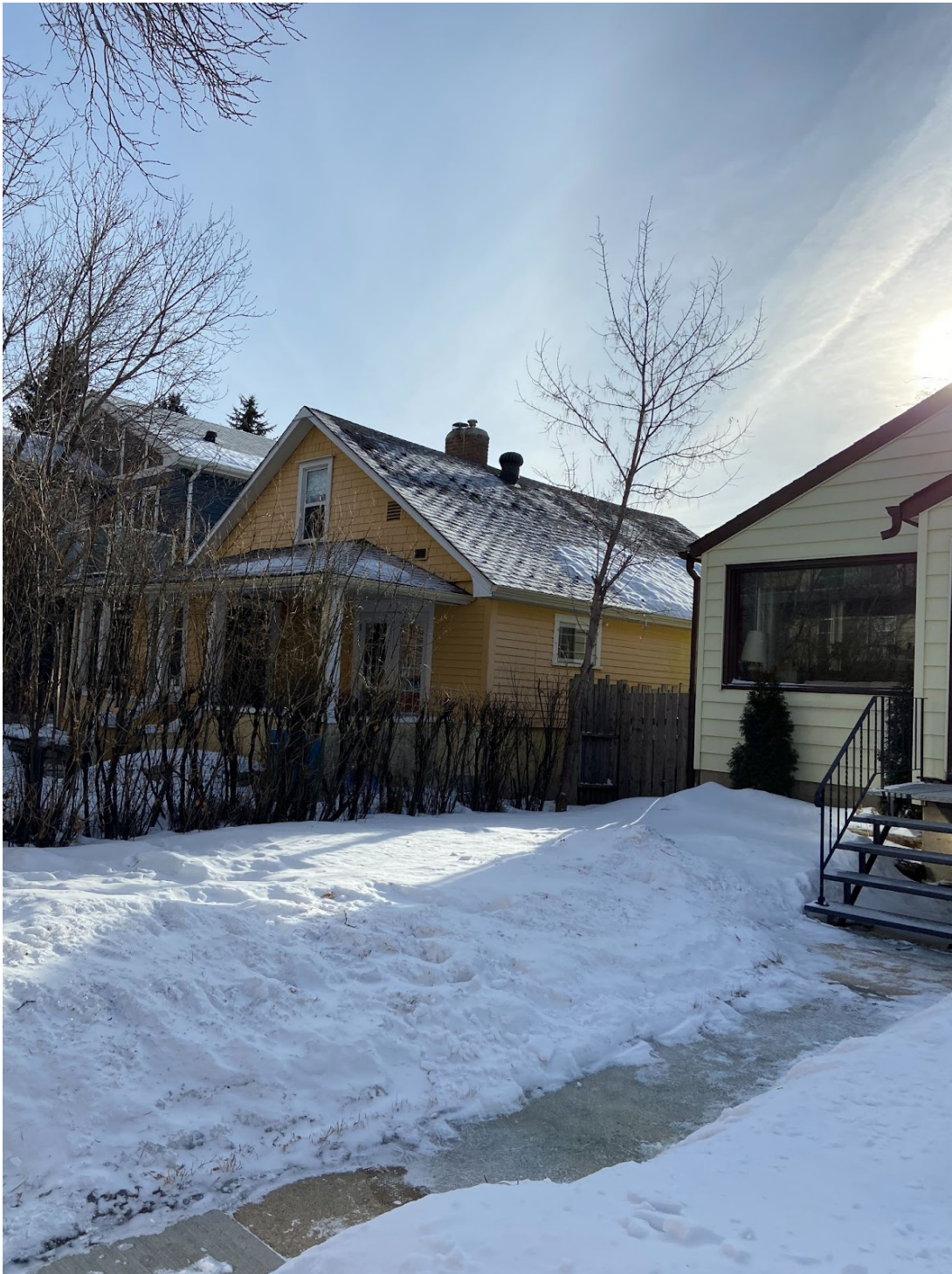
West and north (front) elevations, looking southeast.
