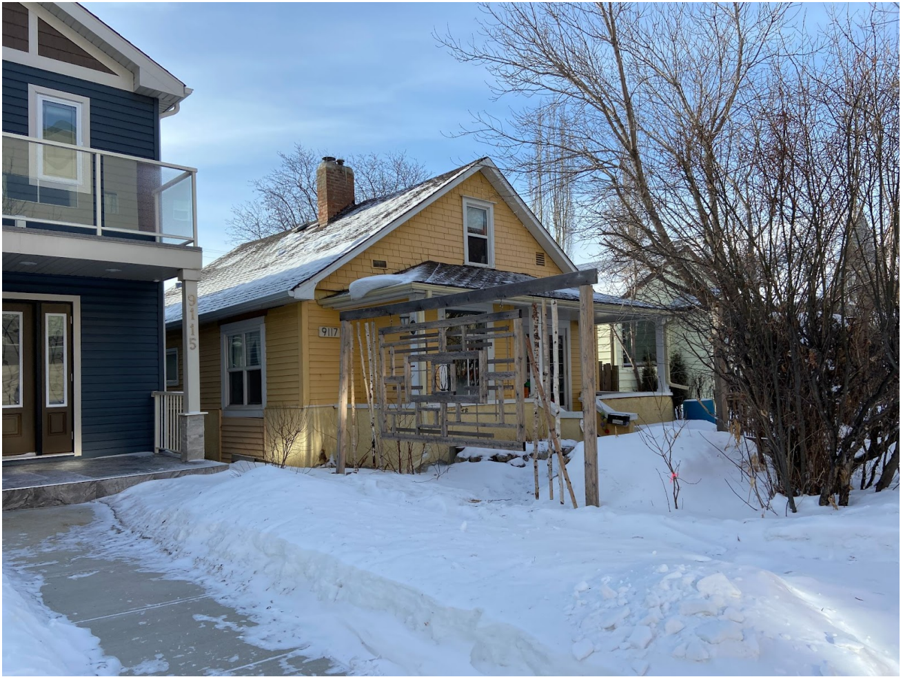
East and north (front) elevations, looking southwest.
