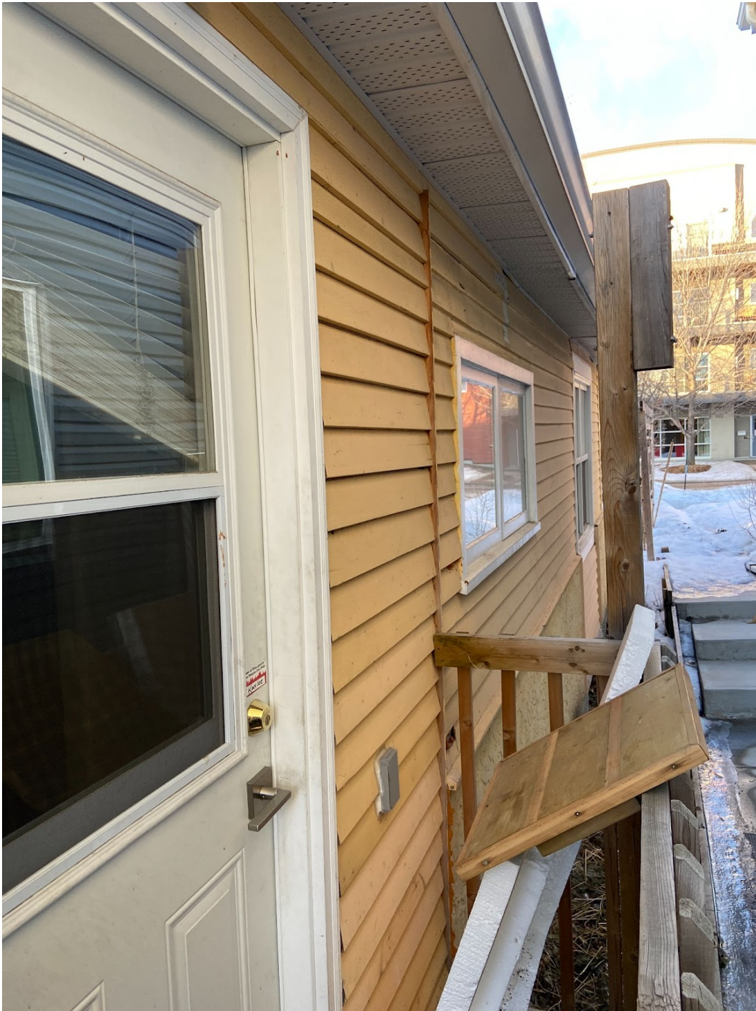
Detail of east elevation, looking north.
