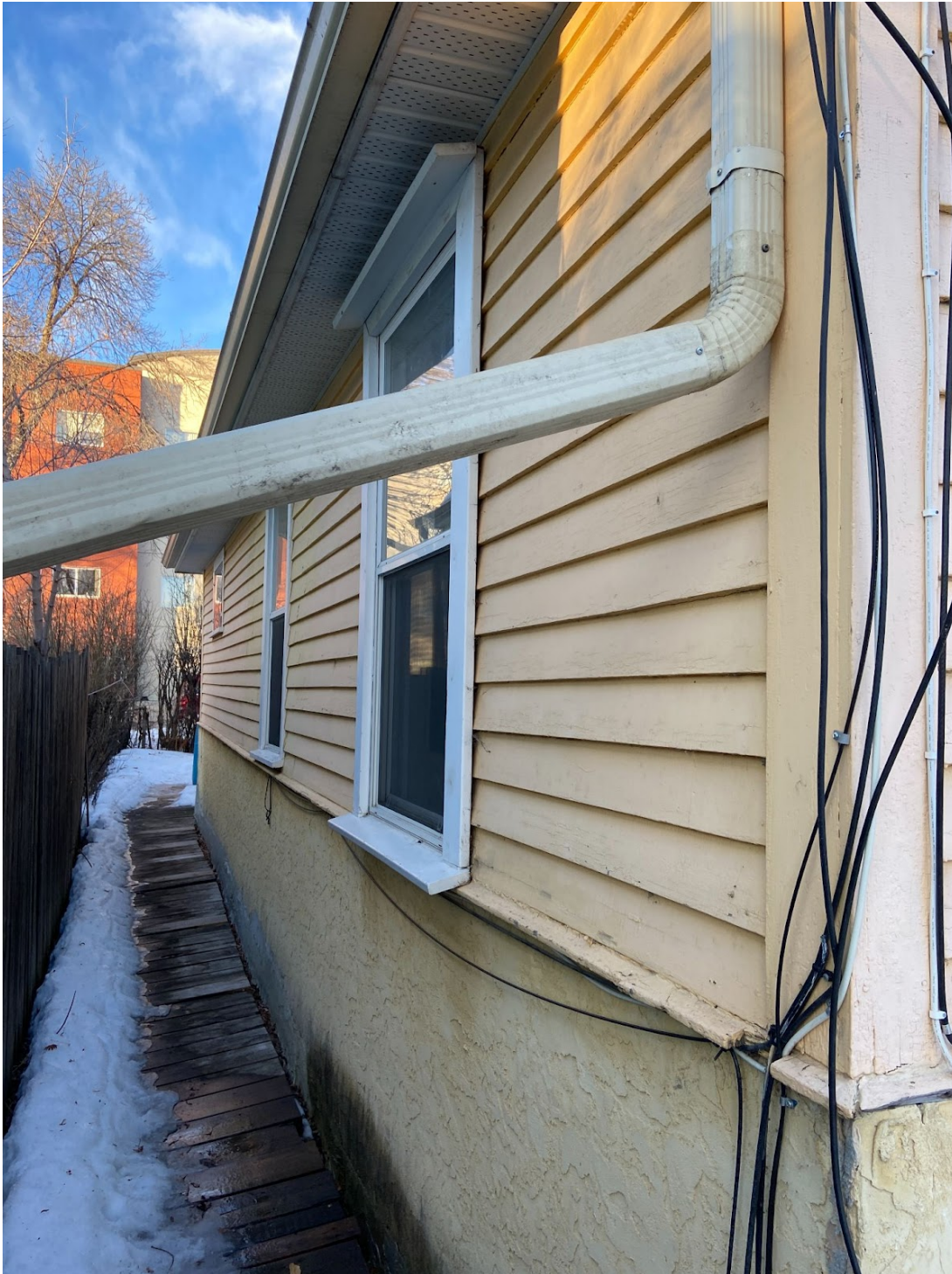
Detail of west elevation, looking north.
