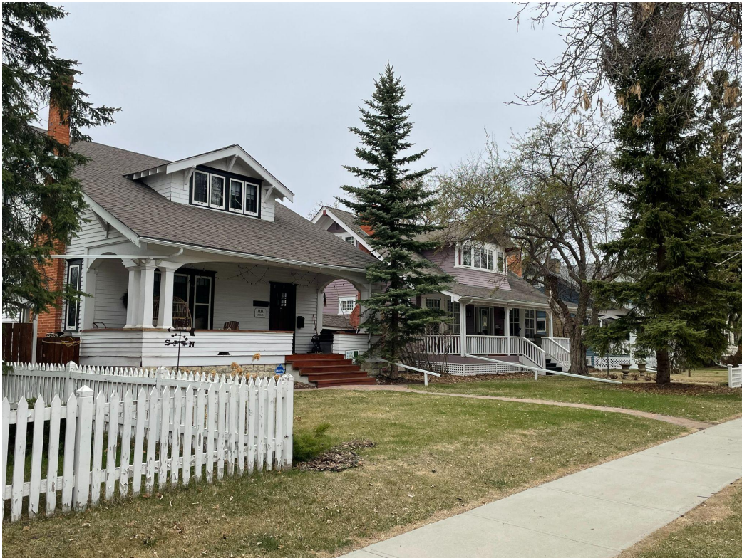
Context photo with Stein Residence in foreground - looking northwest
