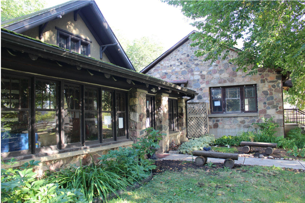
Stone House north elevation, with Keillor Cabin in the foreground
