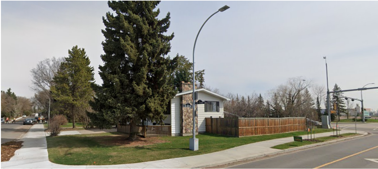
View of the site looking northeast from 63 Avenue NW (Google Street View, May 2022)
