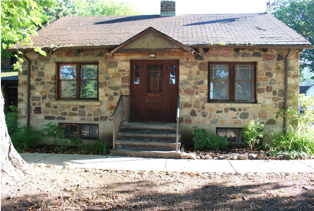
Stone House west (front) elevation
