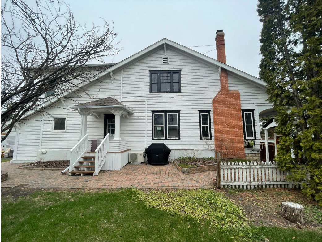
South (side) elevation - looking north
