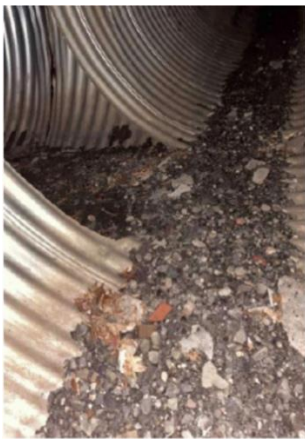
Debris found in Stormwater pipes.
