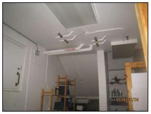
Photograph 20: Pipe wrap labelled "asbestos" in the basement of the John Janzen Nature Centre.
