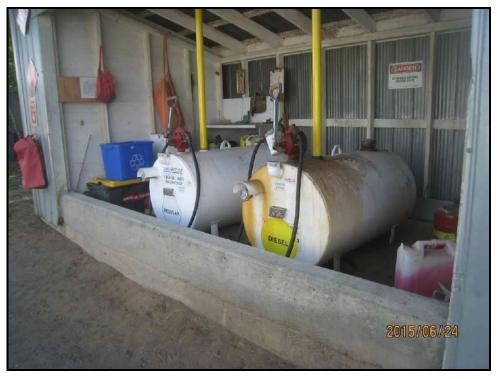
Photograph 12: Fuel ASTs present within the maintenance yard, with some staining noted on the diesel AST.
