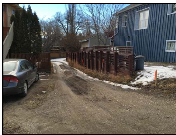
IMAGE OF ALLEY LOOKING SOUTH AND SHOWING ENCROACHMENT DUE TO INSUFFICIENT TURNING RADIUS.
