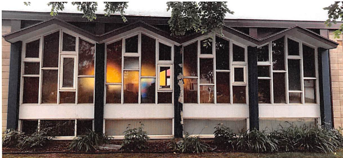
South Elevation - Coloured Glass Windows to the Sanctuary
