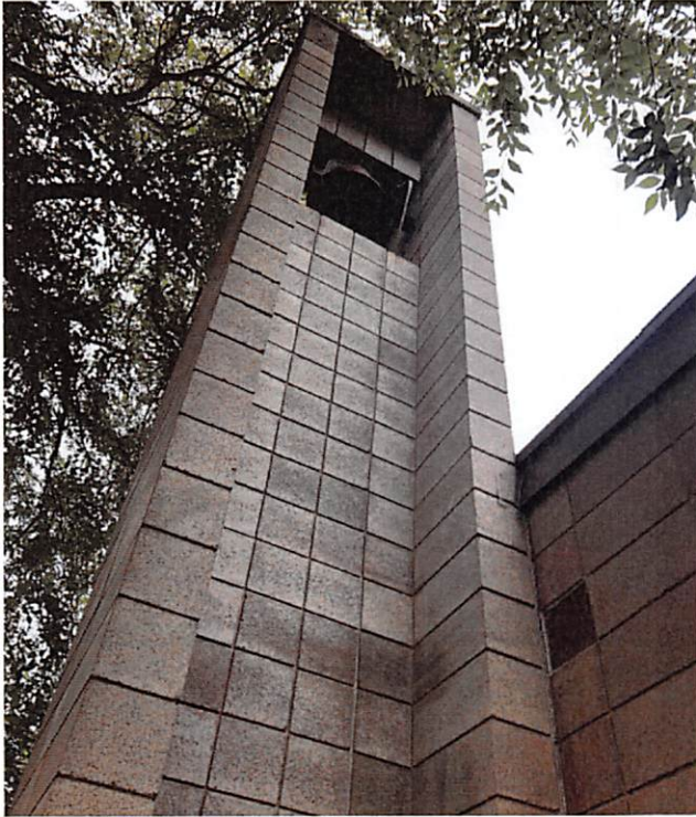
Concrete Block Belltower
