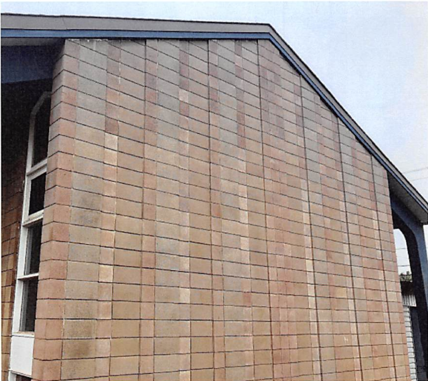
East Elevation - Concrete Block Masonry Units Arranged to Create Patterns and Textures
