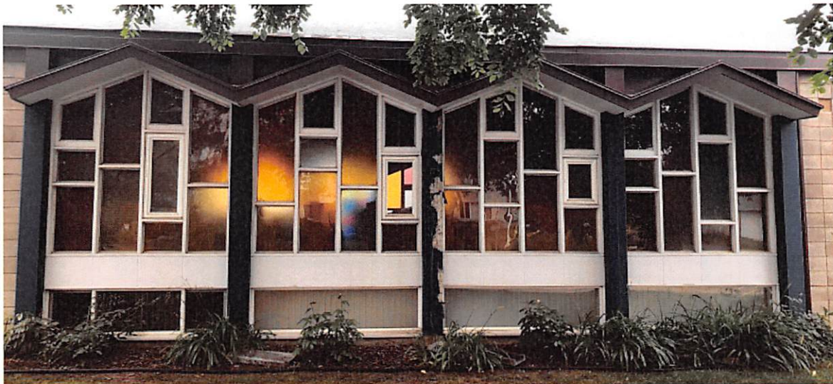
South Elevation - Coloured Glass Windows to the Sanctuary
