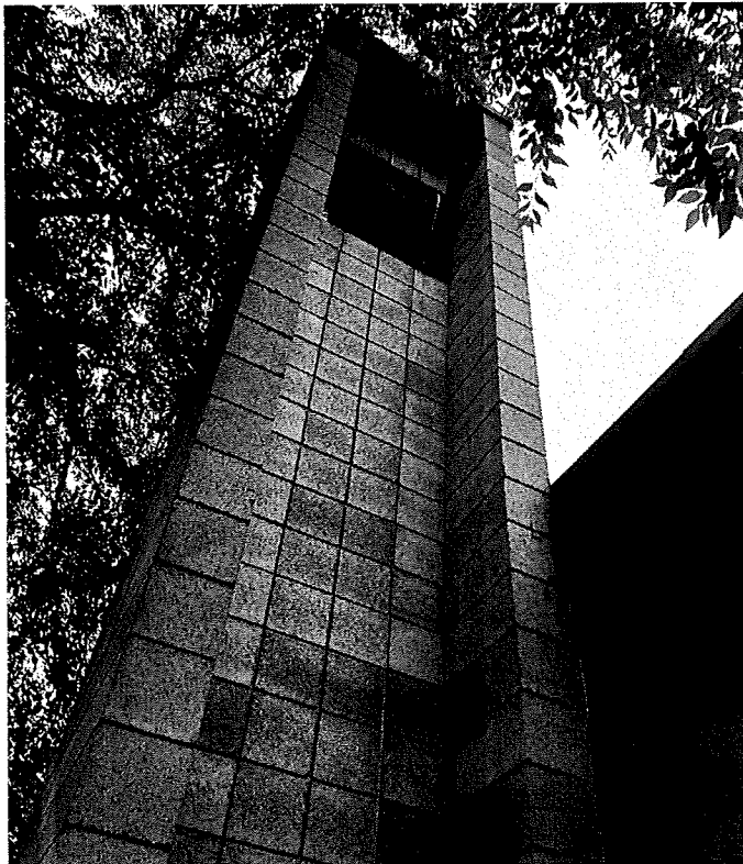
2022 - Concrete Block Belltower
