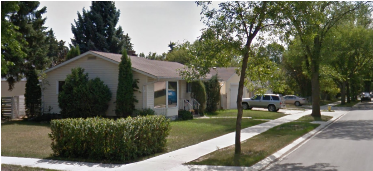
View of the site looking southeast from 106A Avenue NW and 144 Street NW (Google Street View, August 2015)
