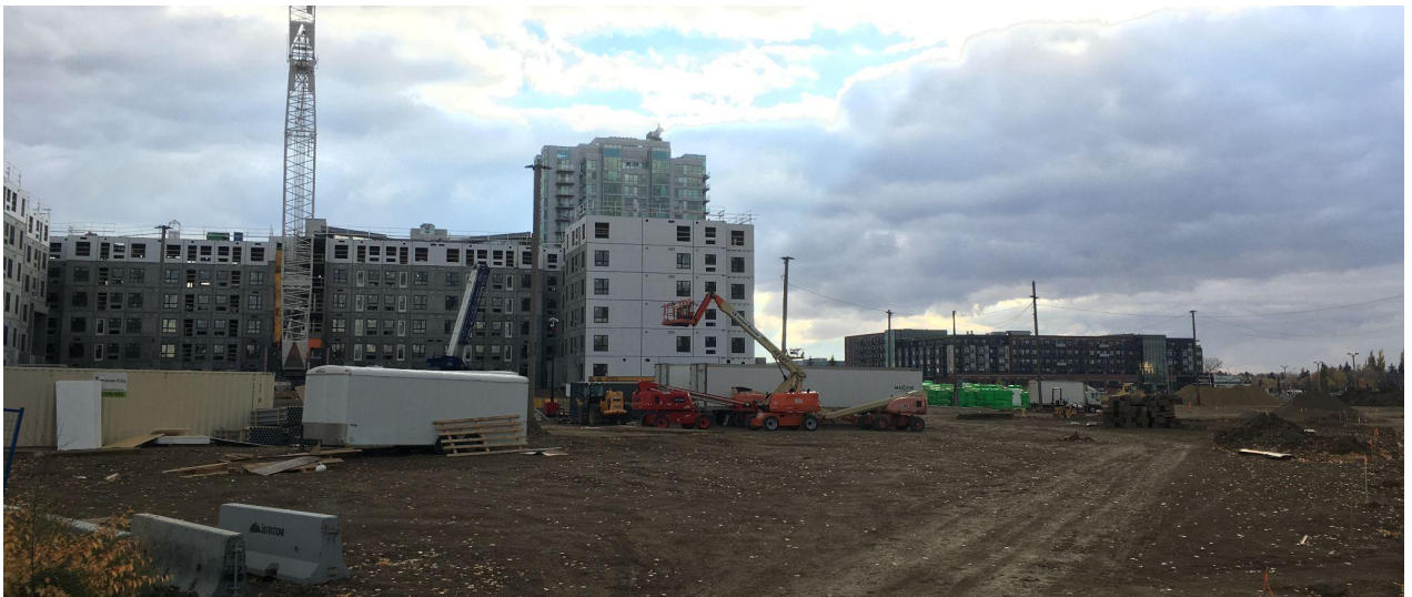
View of the site looking southwest (Century Park Gardens under construction)
