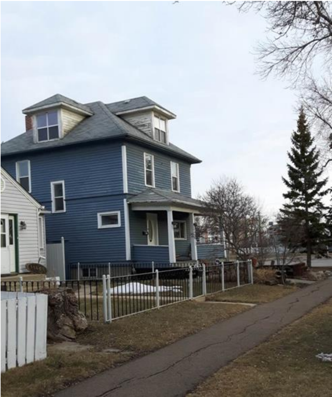
Barto Residence, 2016 – West and North Elevations
