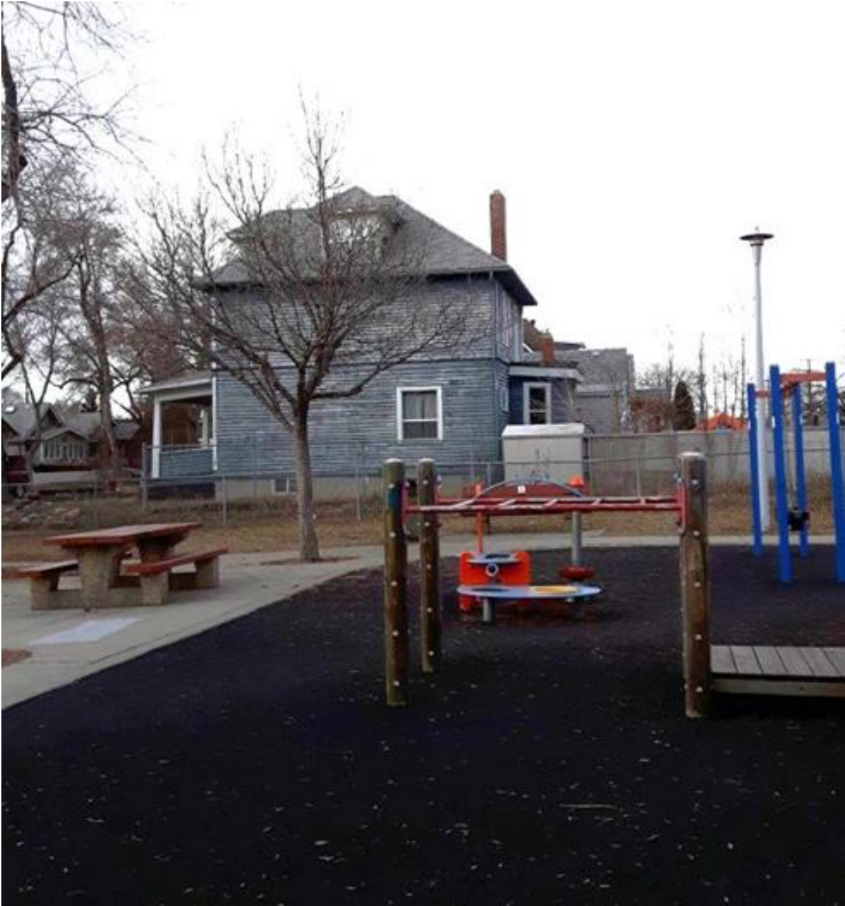
Barto Residence, 2016 – South Elevation
