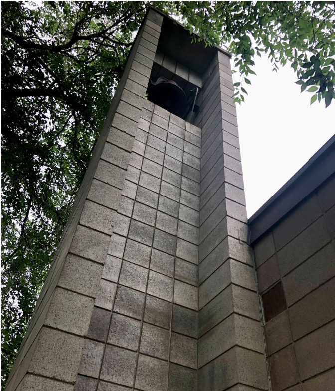
2022 - Concrete Block Belltower
