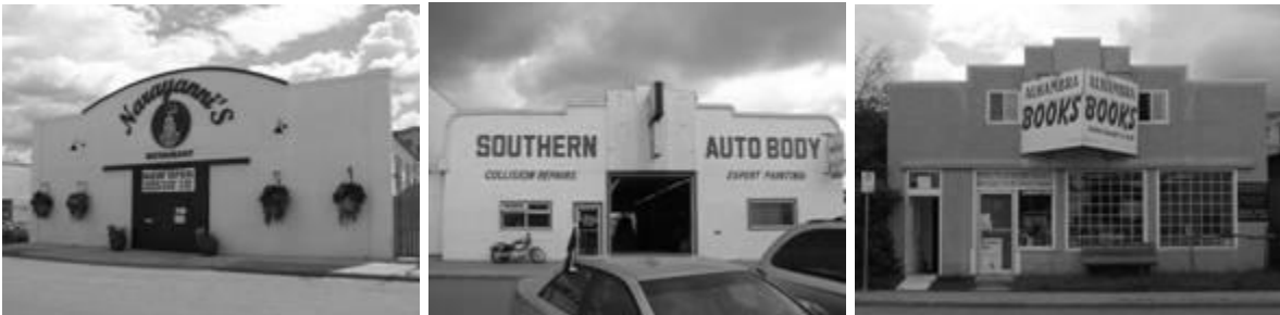
Figure B. False Façades in West Ritchie
