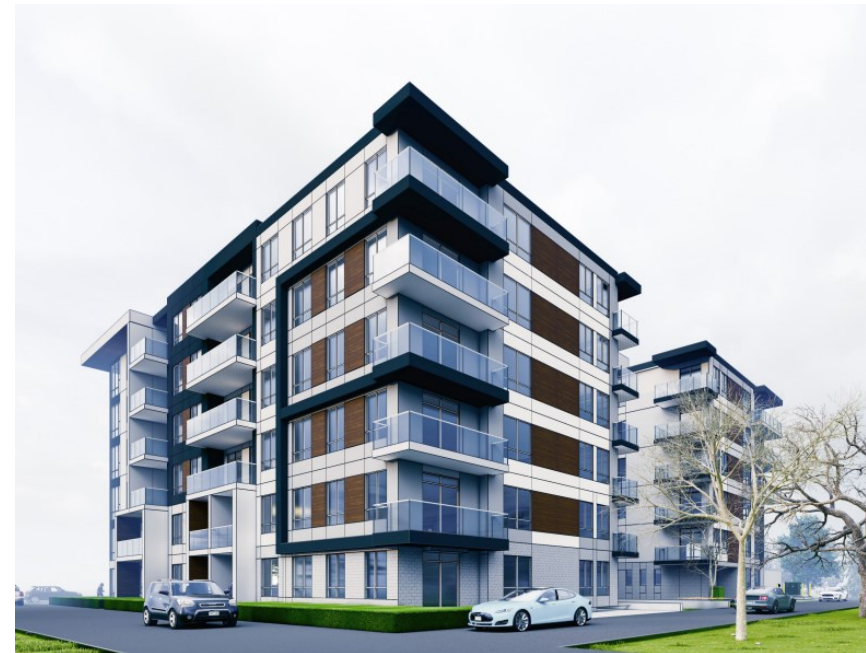
G4 - Southeast view looking northwest
