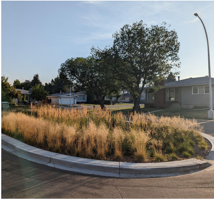
Low Impact Development (LID) Rideau Park, 43 Avenue - 109 Street
