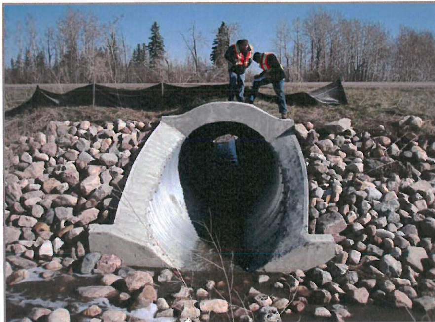
Looking North (Downstream) Through Culvert 402.
