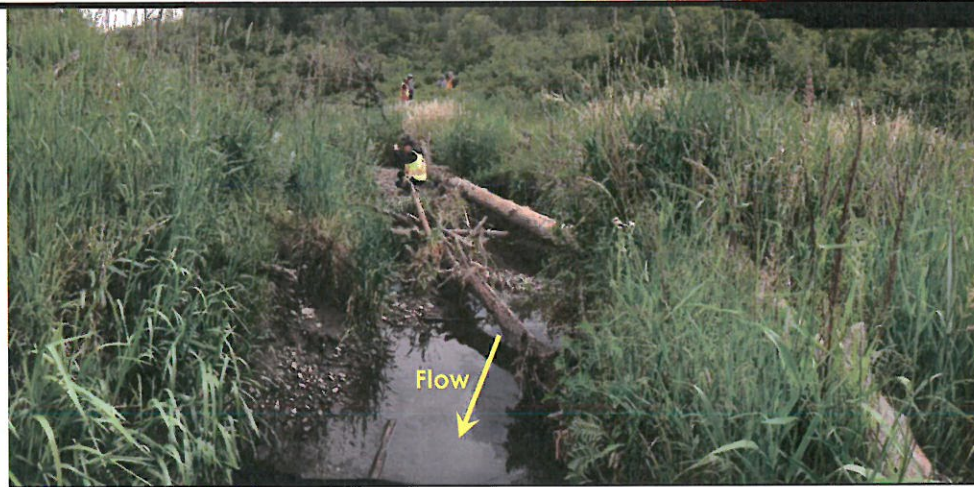
Photo 2: Looking upstream (south) from downstream of crossing. Note debris.
