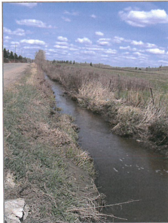
Existing Ditch from Culvert 436 to Culvert 402. Looking Downstream (North) of Culvert 436.
