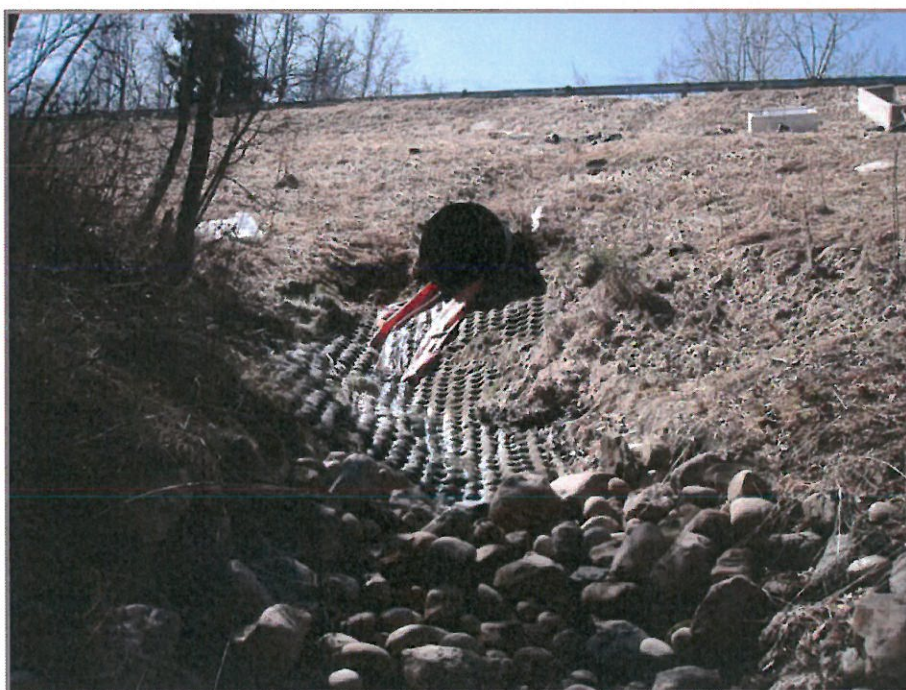
Aurum Creek Downstream of Culvert 5.
