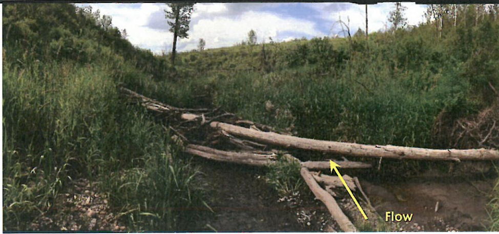
Photo 1: Looking downstream (north) from downstream of proposed crossing. Note debris.
