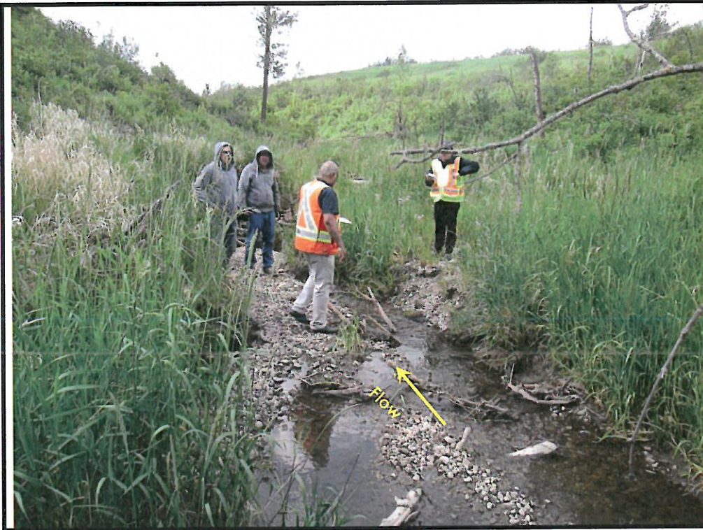
Photo 9: Looking downstream at existing watercourse in vicinity of crossing.
