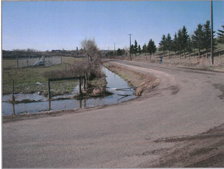
Existing Ditch from Culvert 436 to Culvert 402. Looking Upstream (South) of Culvert 402.
