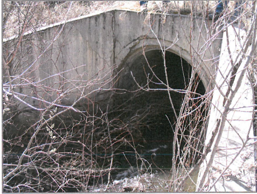
Culvert C8-2 Inlet.
