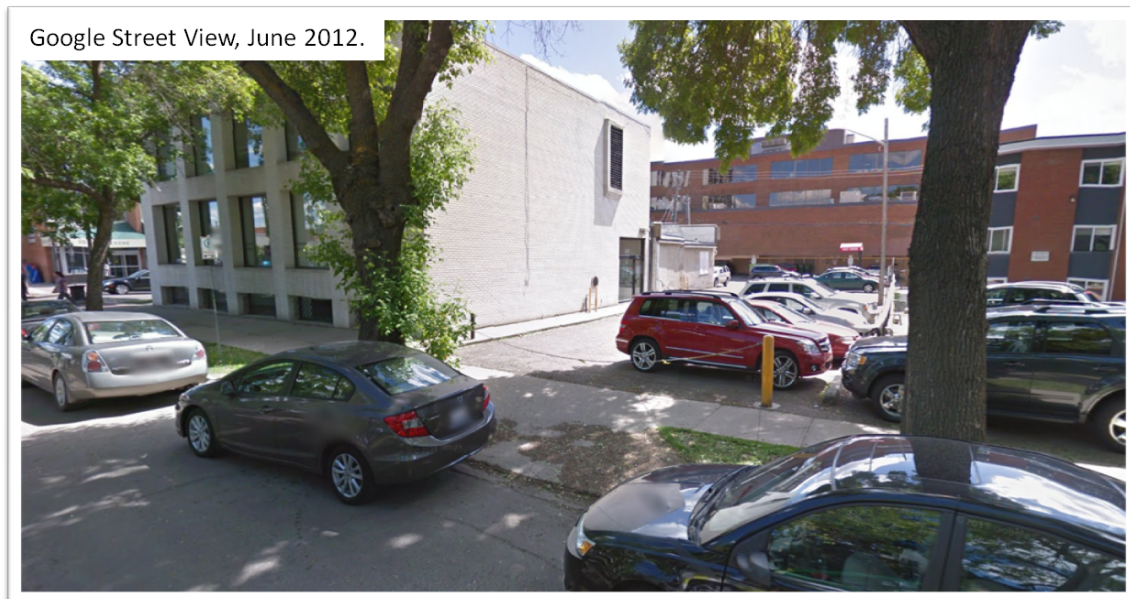
Figure 2. Google Street View Image of 8230 105 Street NW
