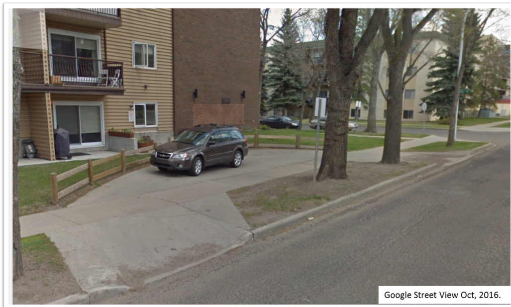
Figure 2. Google Street View Image of 10208 113 Street NW
