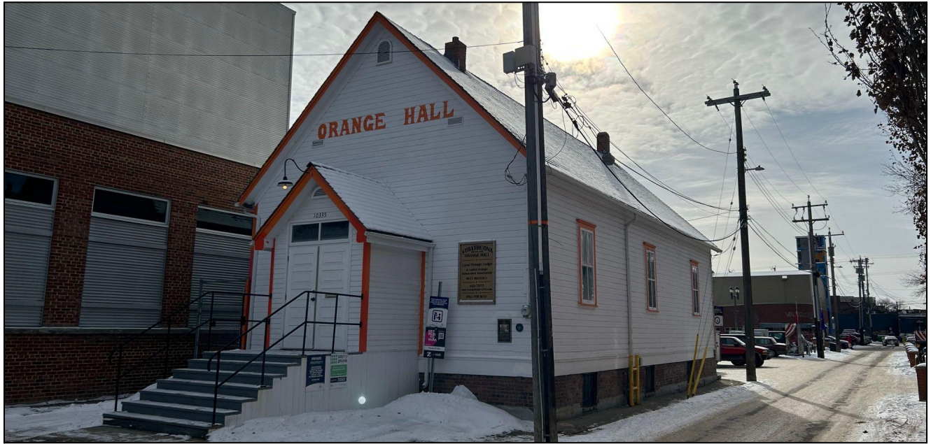
View of the Orange Hall looking southeast from the lane
