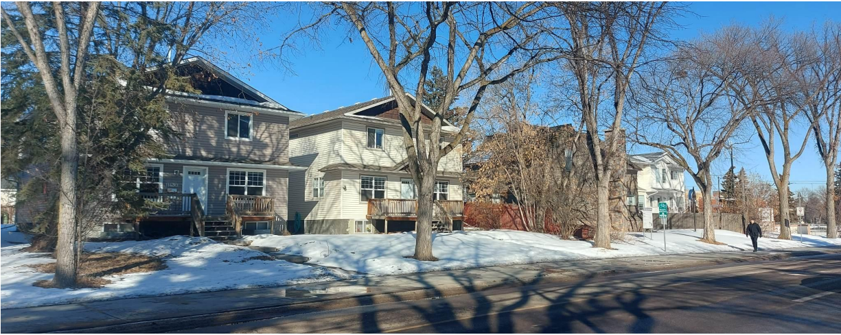
View of the site looking northeast from 76 Avenue NW
