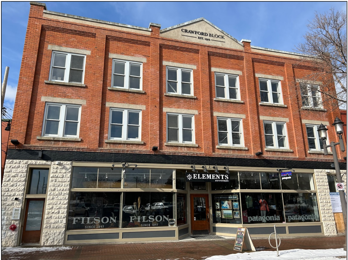
View of the historic 1912 Crawford Block looking west from Gateway Boulevard NW
