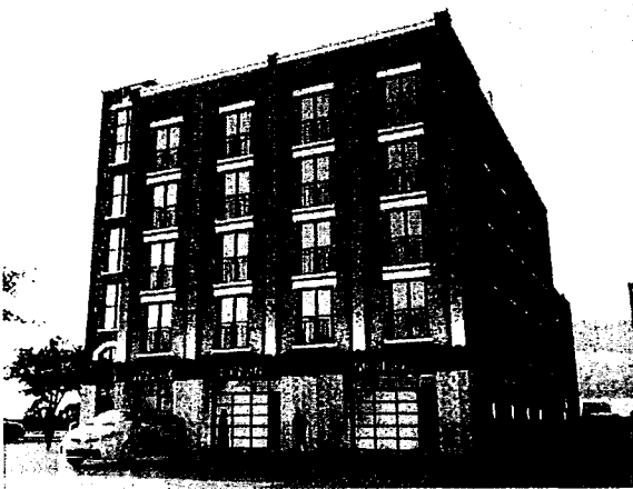
VIEW OF SOUTHWEST CORNER OF BUILDING ALONG THE LANES
