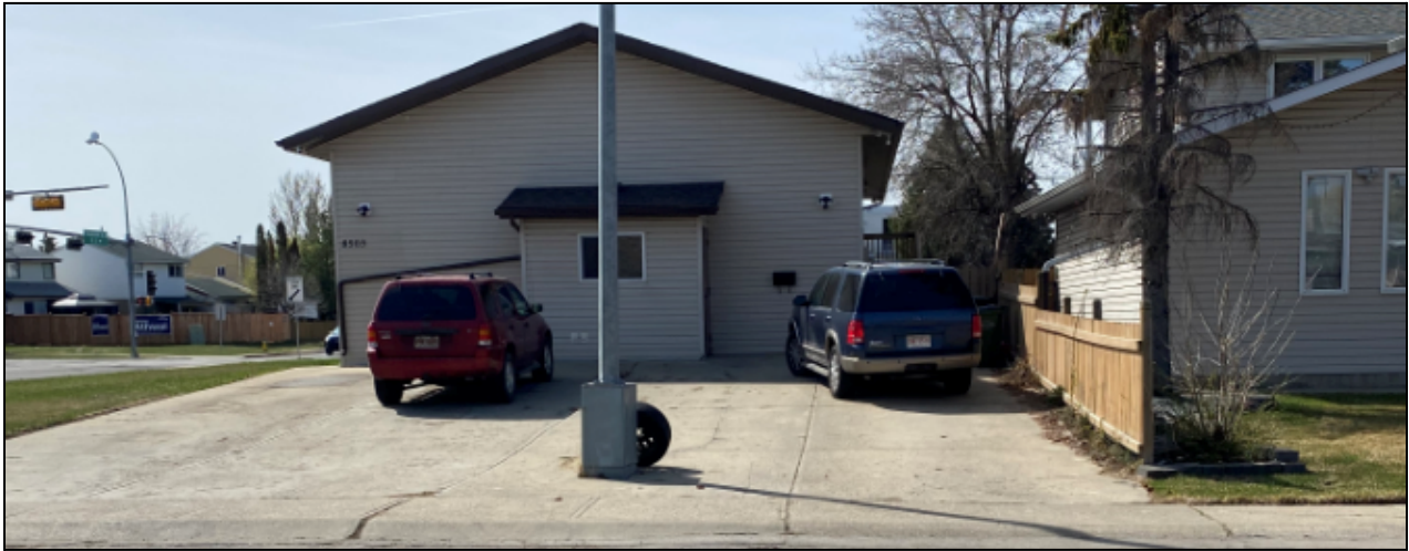
View of the site looking south from 39A Avenue NW.
