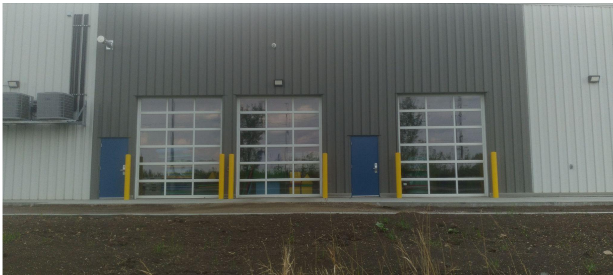
View of the building looking south from the Shared Use Path on south side of 137 Avenue NW
