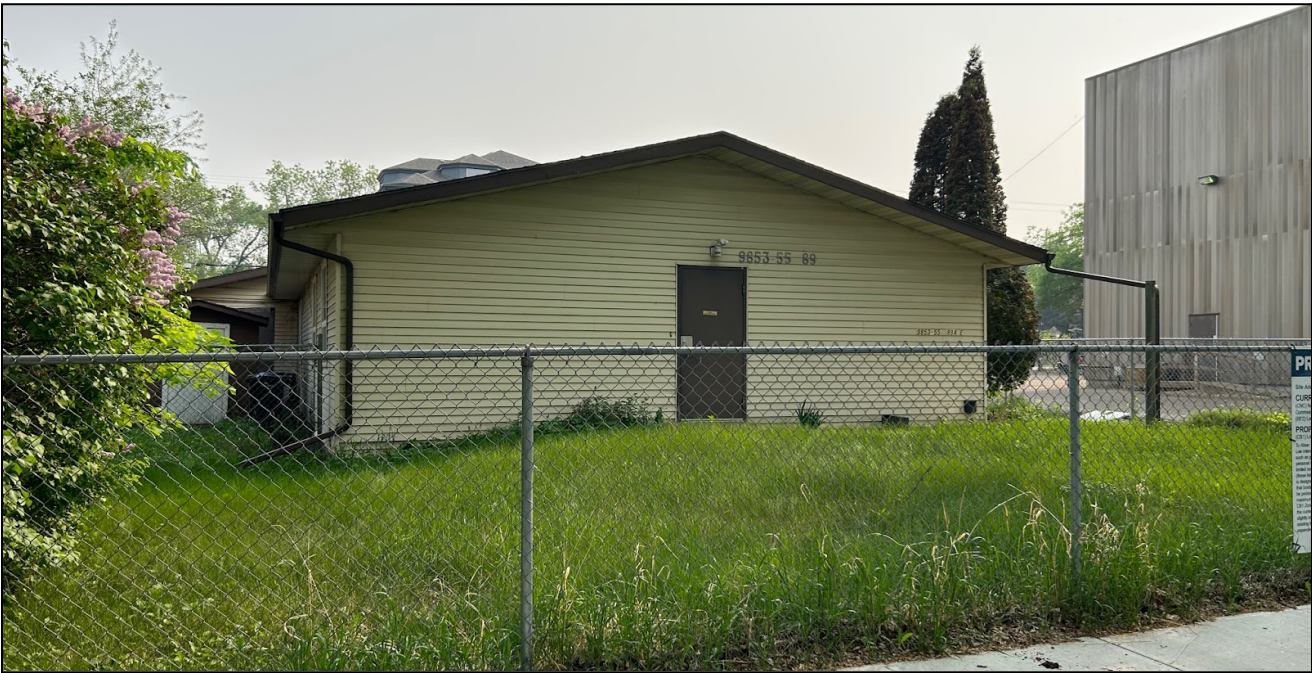
View of the site looking south from 89 Avenue NW
