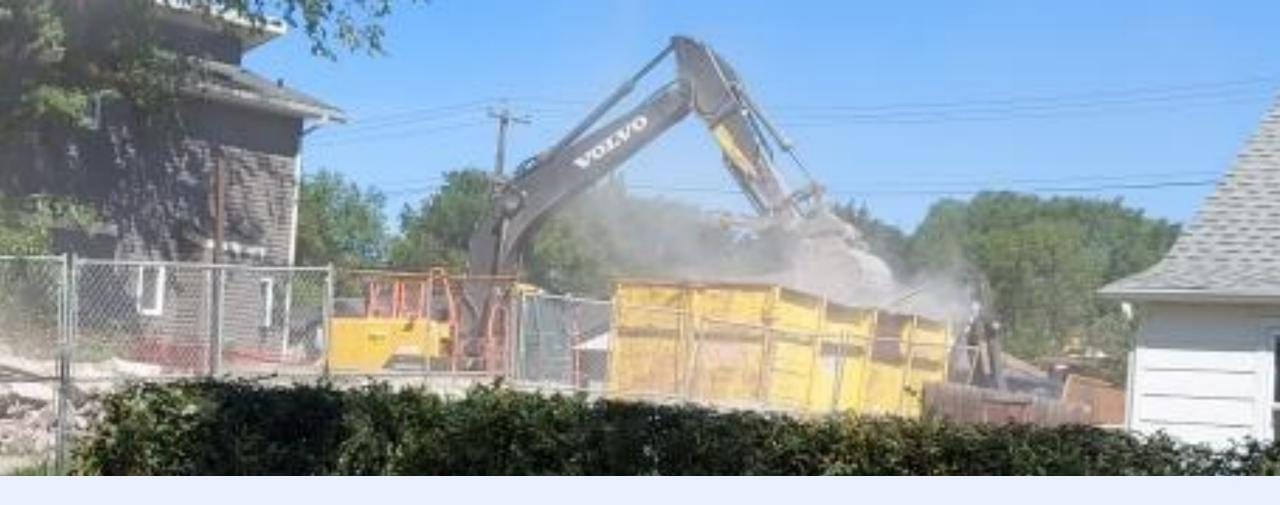
Demolition disturbs lead paint and produces significant emissions of lead dust and other contaminants
