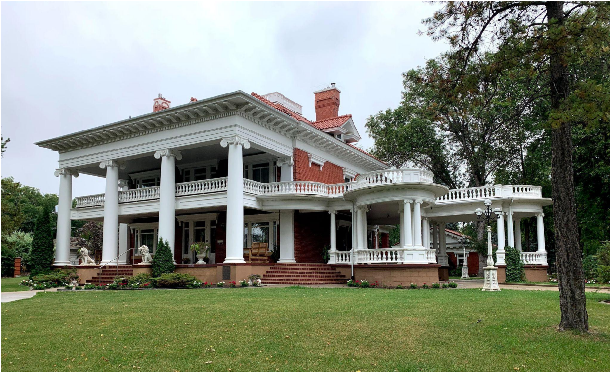
South and East Elevations
