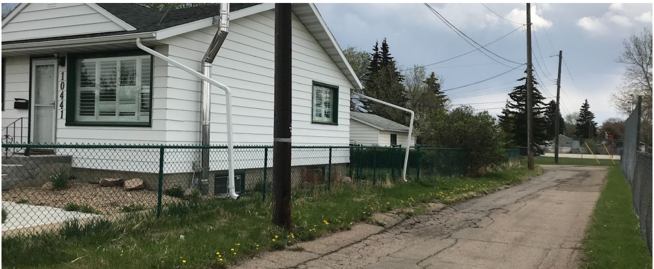
View of the site looking northeast from the southern lane
