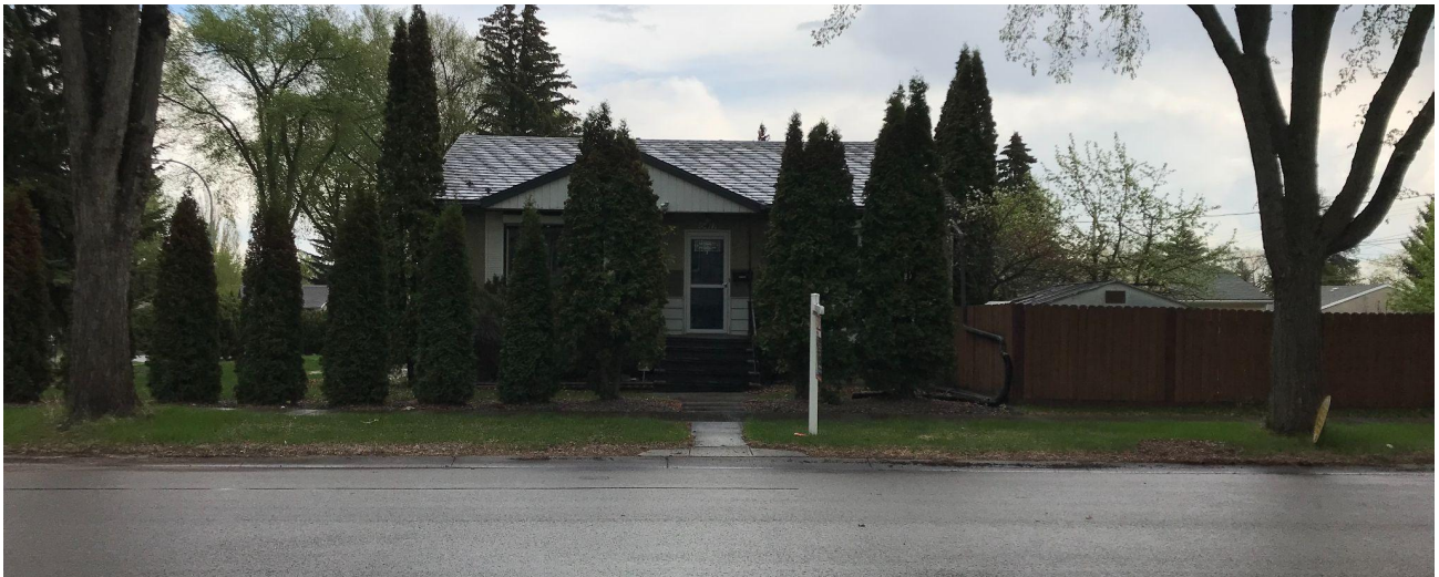
View of the site looking east from 93 Street NW
