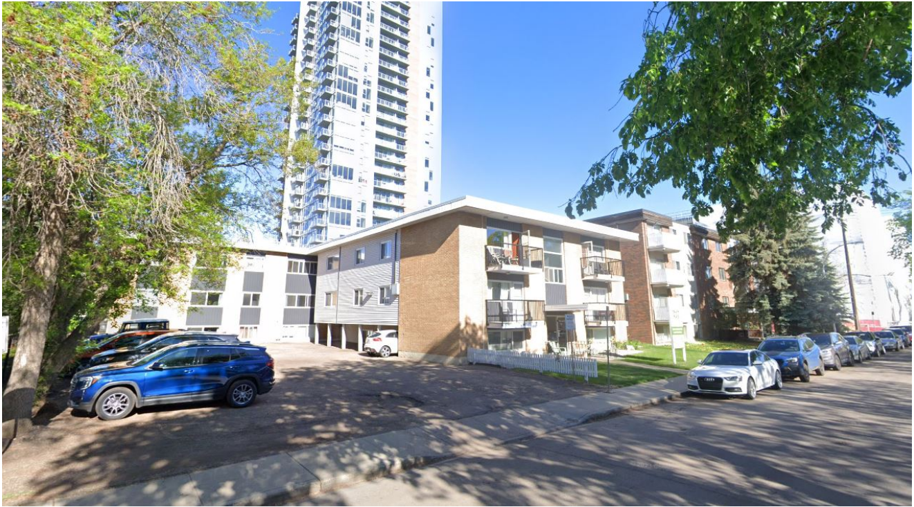
View of the site looking northwest from 123 Street NW
