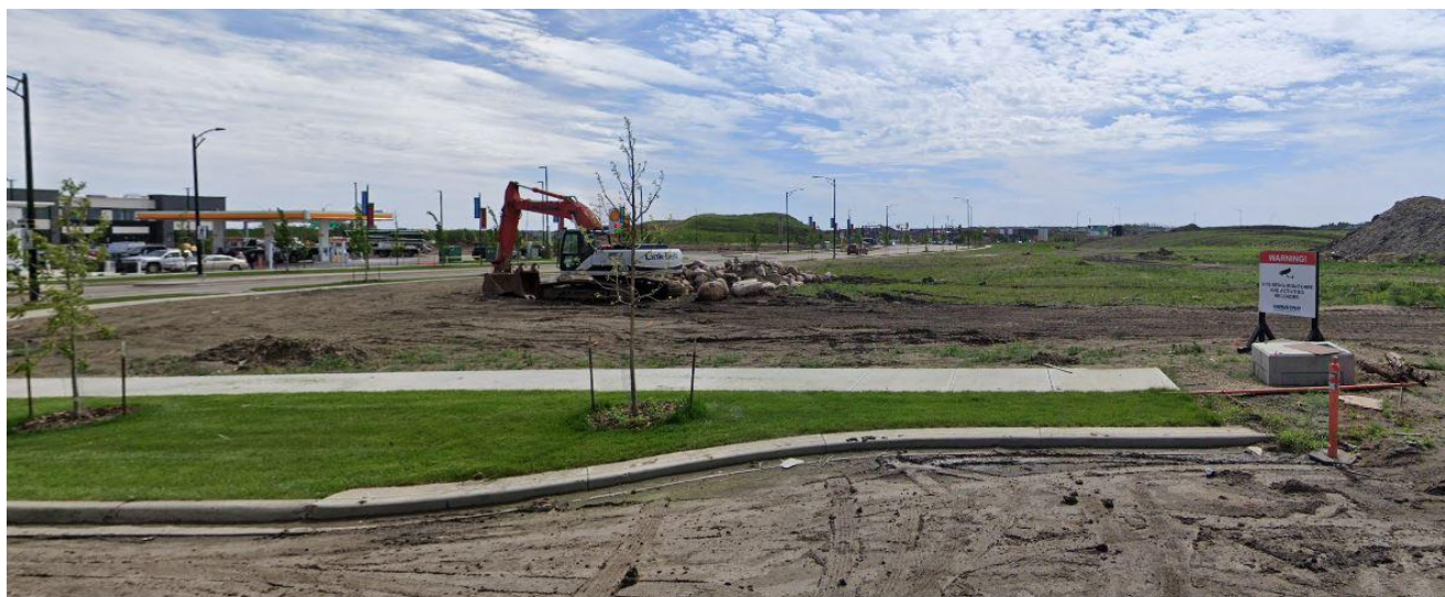
Figure 2 - View of the site looking east from 69A Street NW
