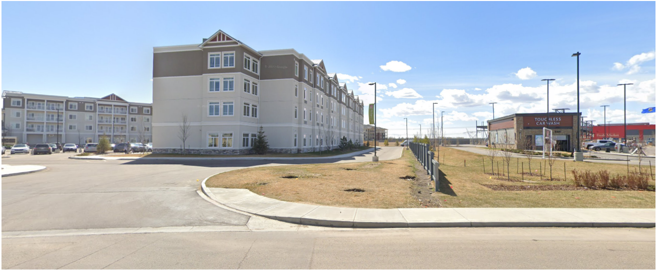
View of the site entrance looking south from Mullen Road NW.
