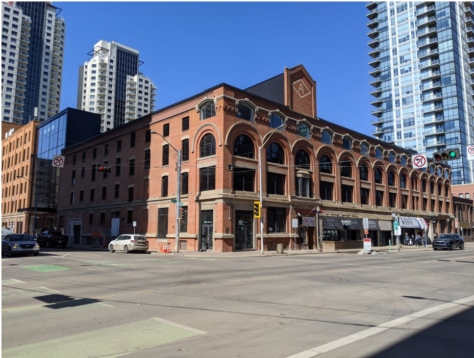
View of east and south elevations, looking northwest from 102 Avenue NW.
