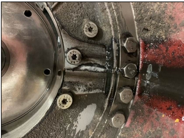
Figure 3: Metal contamination inside the transmission.
