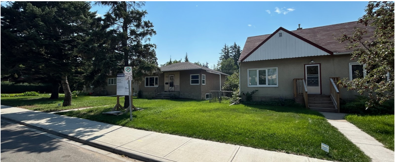
View of site looking southeast from University Avenue NW
