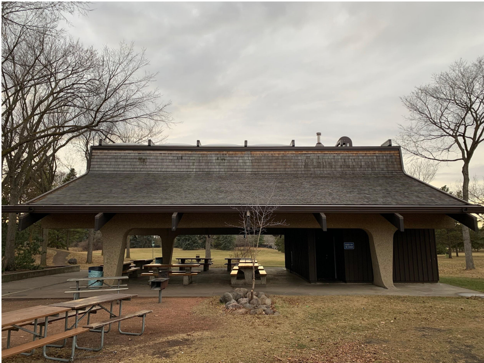
Picnic Shelter #3 east elevation, looking west
