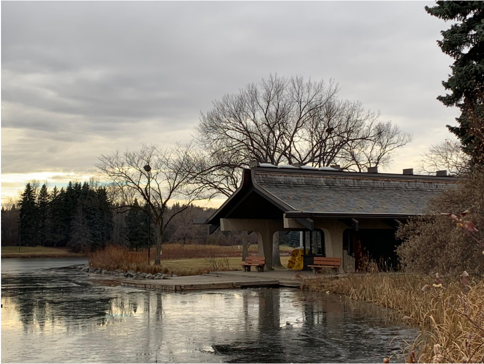
Boat House south elevation, looking northwest
