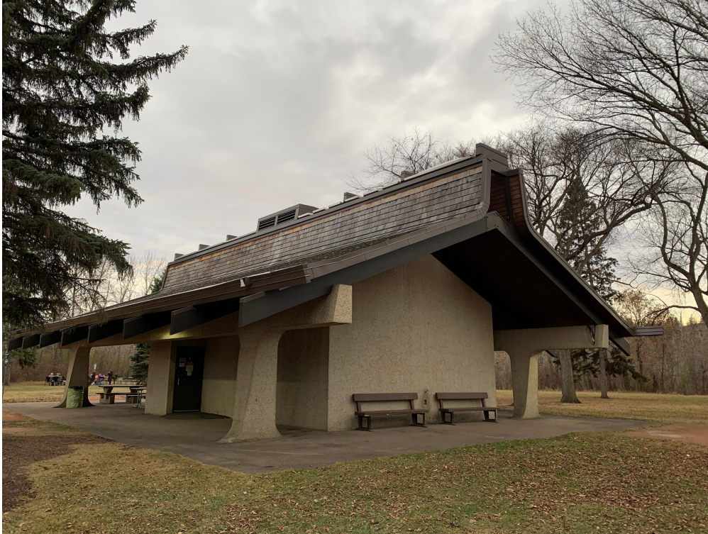
Picnic Shelter #1 north and east elevations, looking southwest
