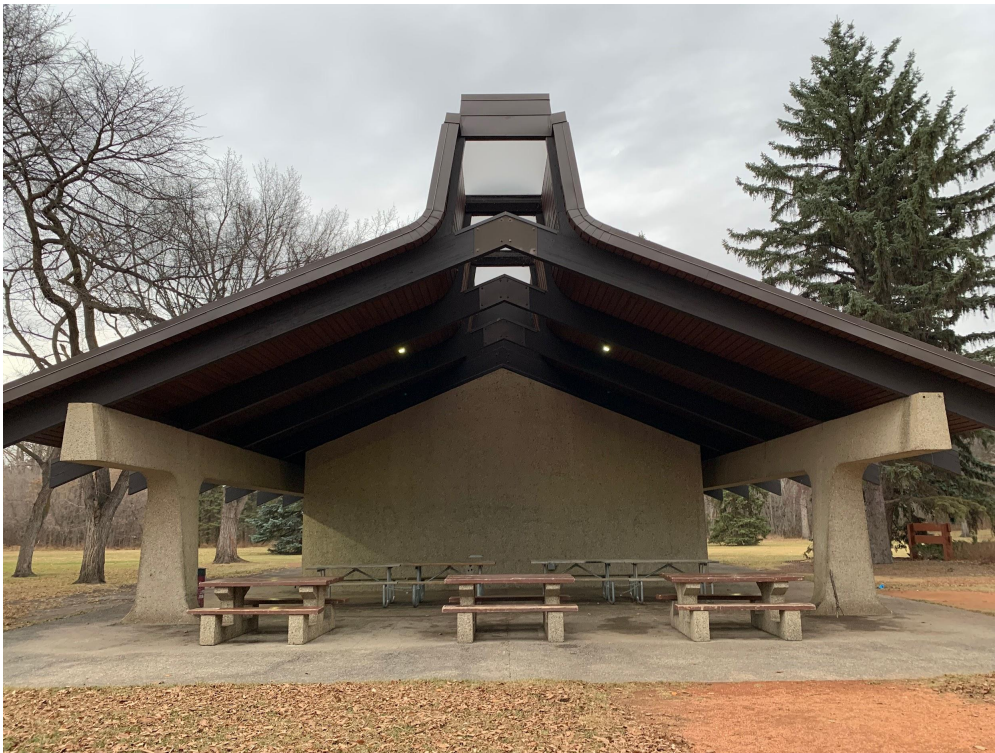
Picnic Shelter #1 south elevation, looking north
