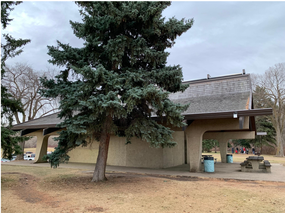
Picnic Shelter #2 west elevation, looking east
