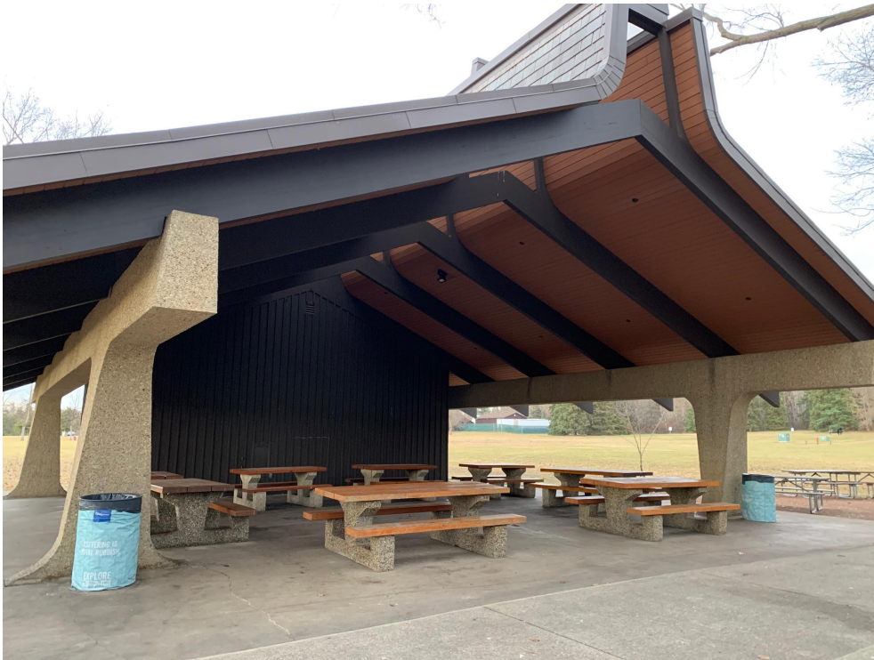
Picnic Shelter #3 south elevation, looking north
