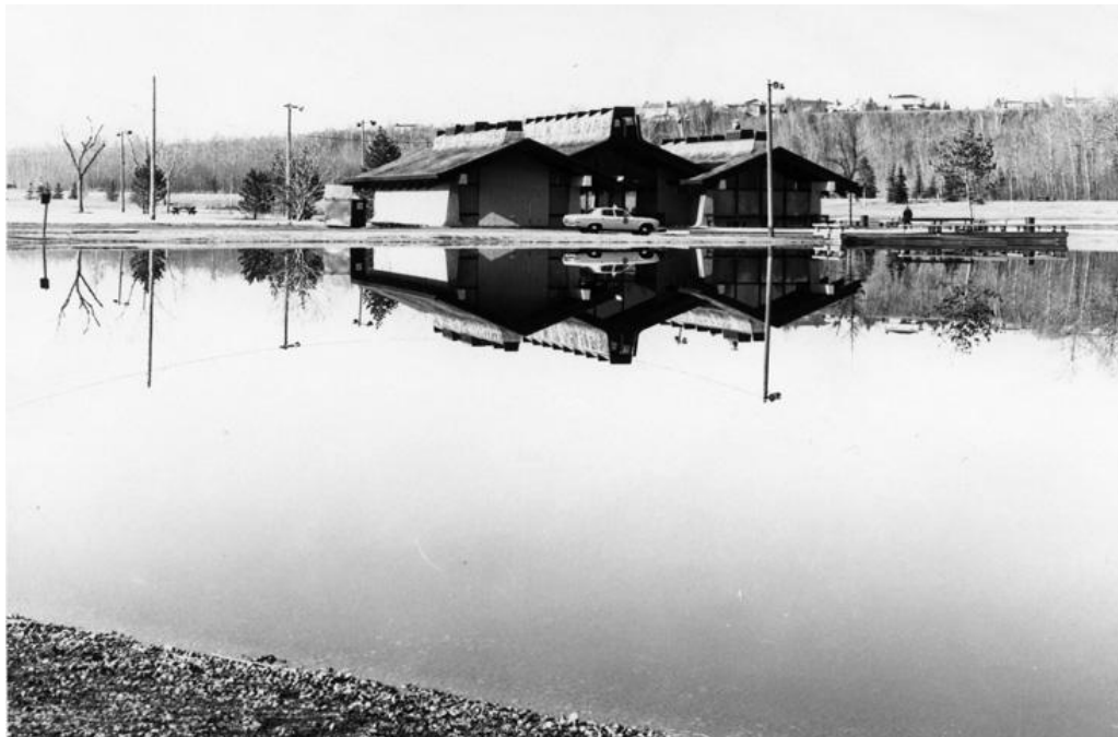
Main Pavilion and lake, 1972 (City of Edmonton Archives, EA-20-6169)
