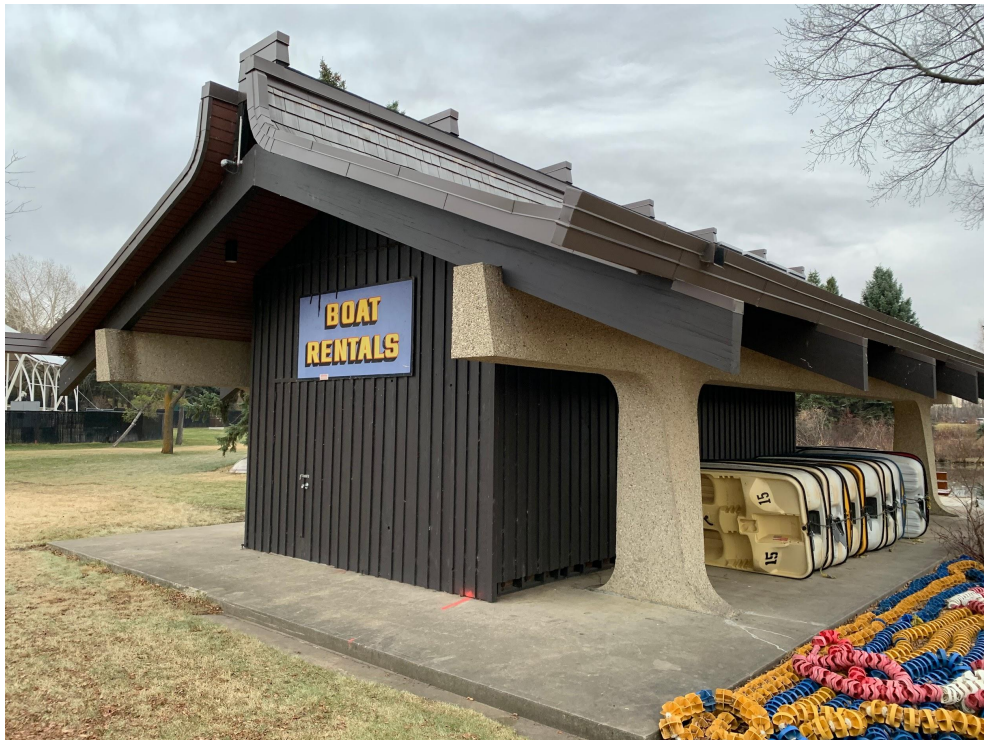
Boat House north and west elevations, looking southeast
