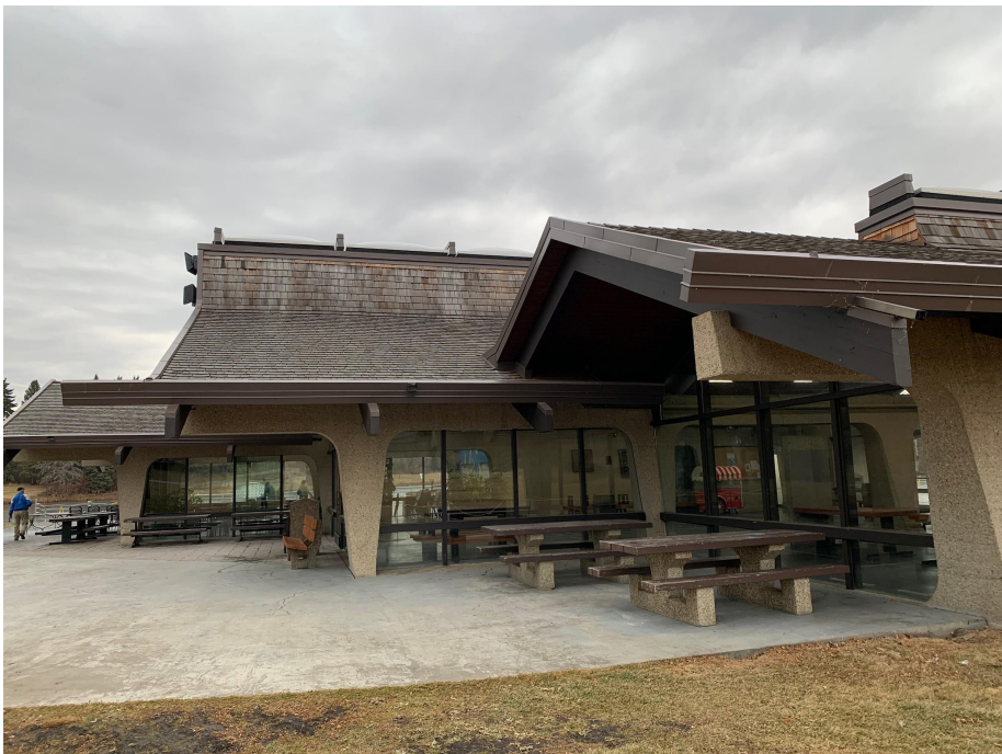
Main Pavilion south entrance, looking west
