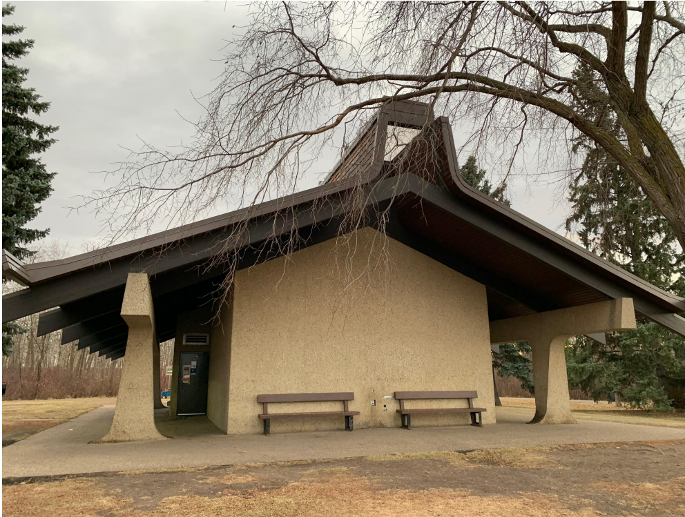
Picnic Shelter #2 north elevation, looking south
