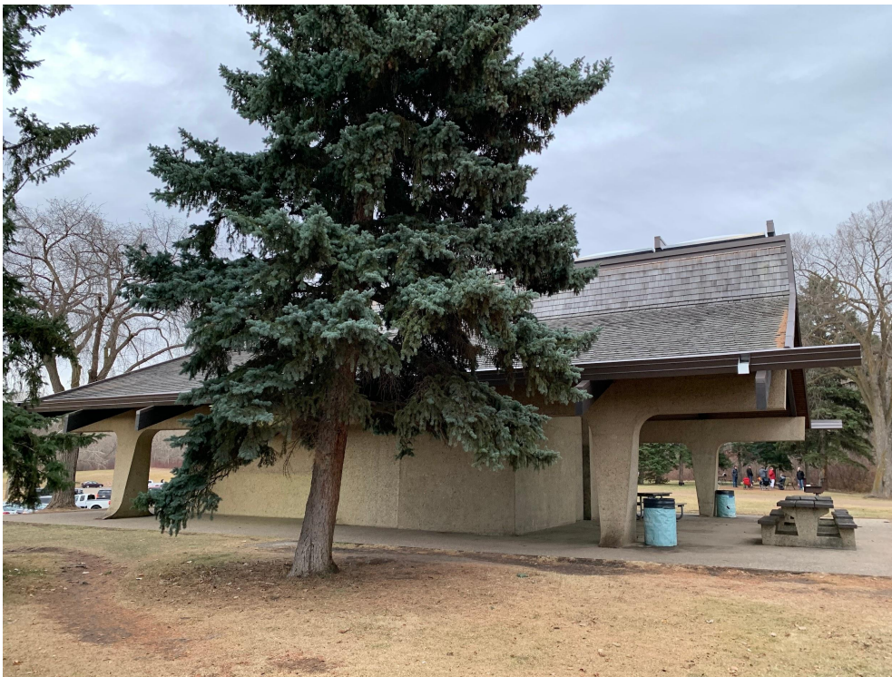
Picnic Shelter #2 west elevation, looking east
