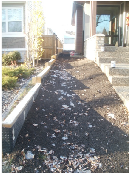
Internal swales are supported by retaining walls with moisture barriers
