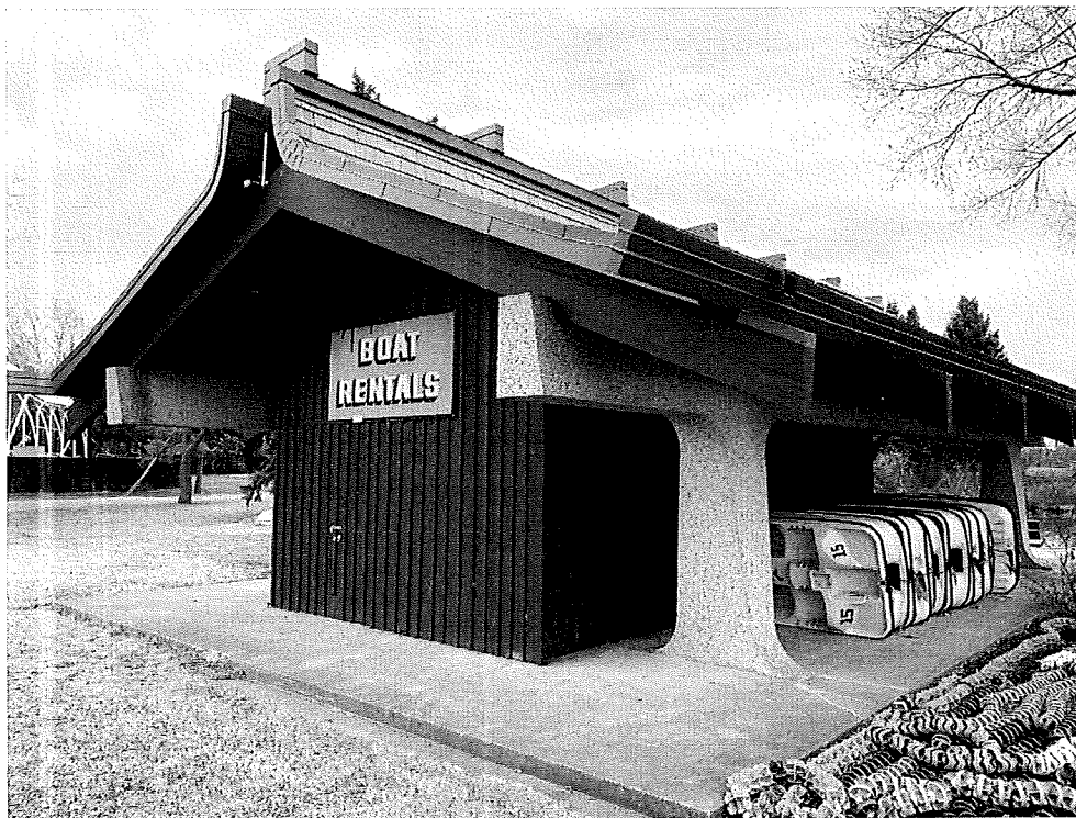
Boat House north and west elevations, looking southeast
